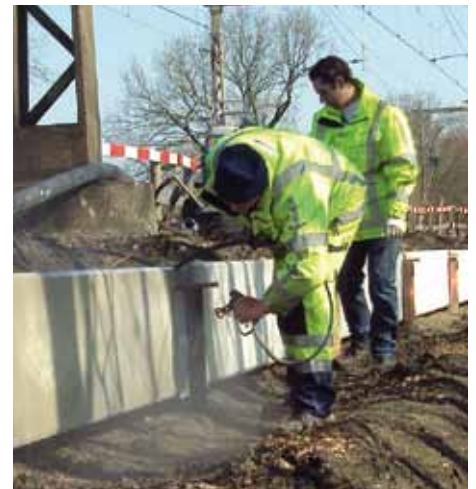
Aanbrengen anti-graffiti coating
